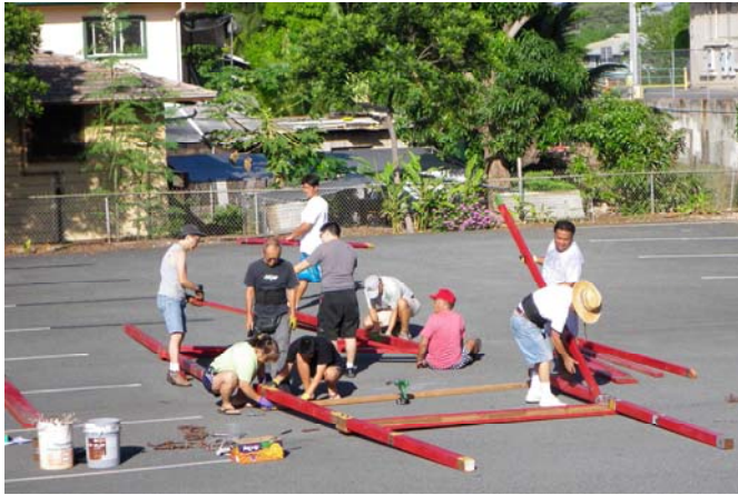
Constructing the Yagura. (more pictures next month)
